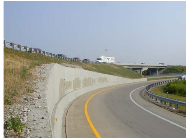
6 – Retaining Wall on I-264 WB to I-64 EB Ramp
