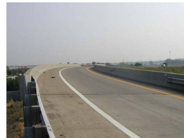
3 – I-64 WB to I-264 WB Ramp Looking at Bridge over I-64
