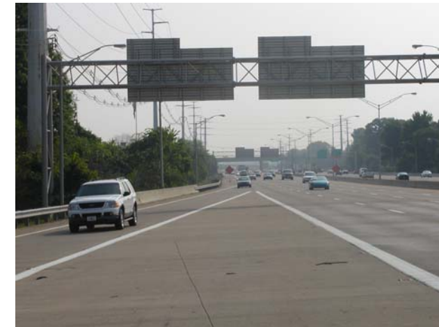
7 – I-264 WB Exit Ramp to Breckenridge Lane Facing East
