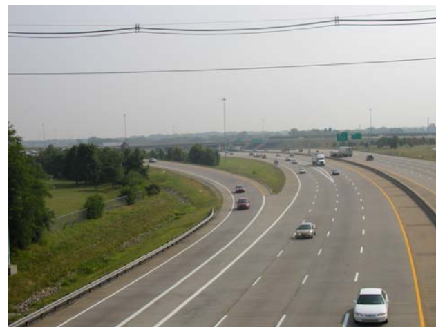
10 – Browns Lane Bridge over I-264 Facing East
