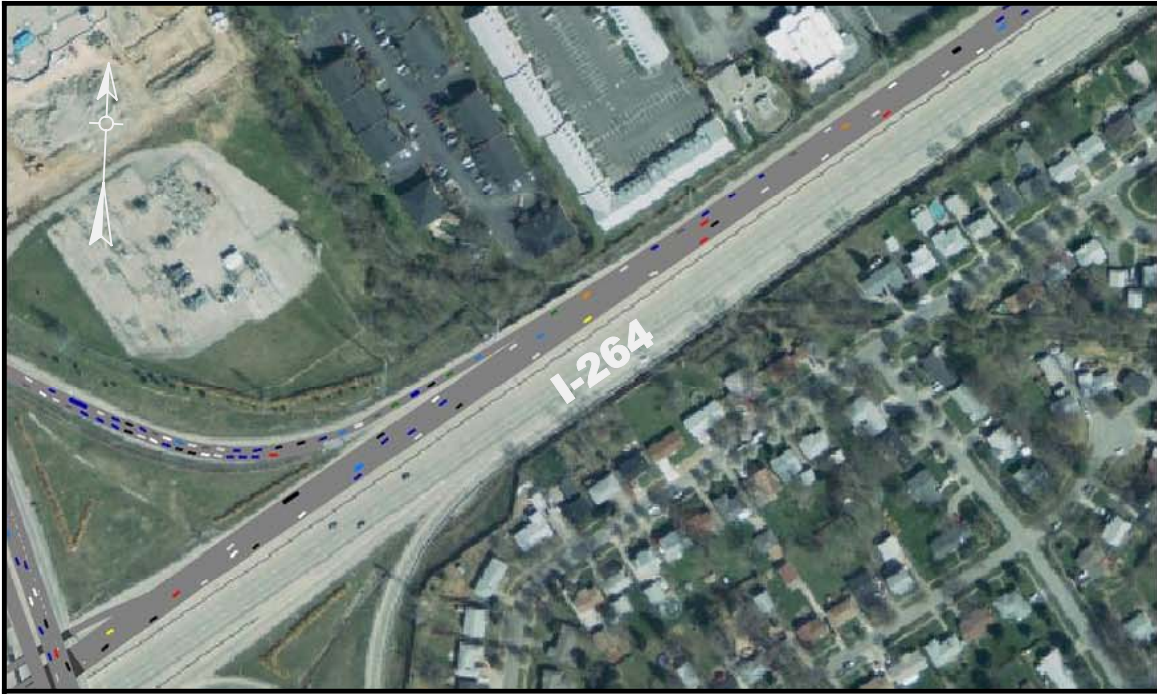
2010 AM - I-264 from I-64 to Breckenridge Lane: Longer queues on exit ramps when compared to 2005 AM scenario.
