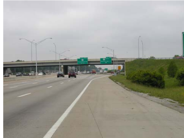
17 – Looking West at Breckenridge Lane Bridge over I-264
