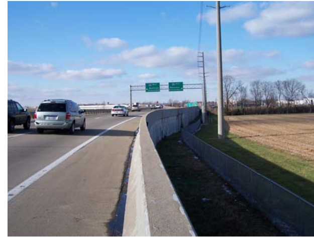
14 – I-64 WB Exit Ramp @ I-264
