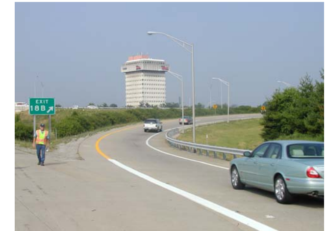
8 – I-264 WB Exit Ramp to Breckenridge Lane Facing West
