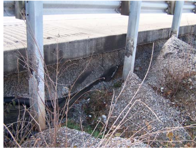
13 – I-64 WB Shoulder West of Oxmoor Farm Road Overpass
