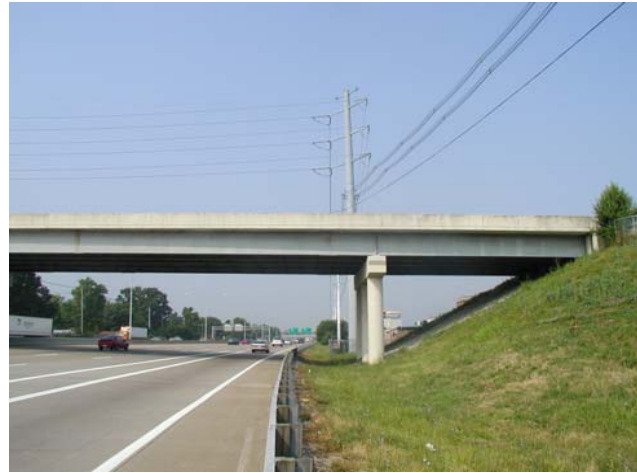
12 – Looking West at Browns Lane Bridge from I-264 WB
