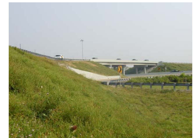
4 – Looking North Towards I-64 WB to I-264 WB Ramp over I-64
