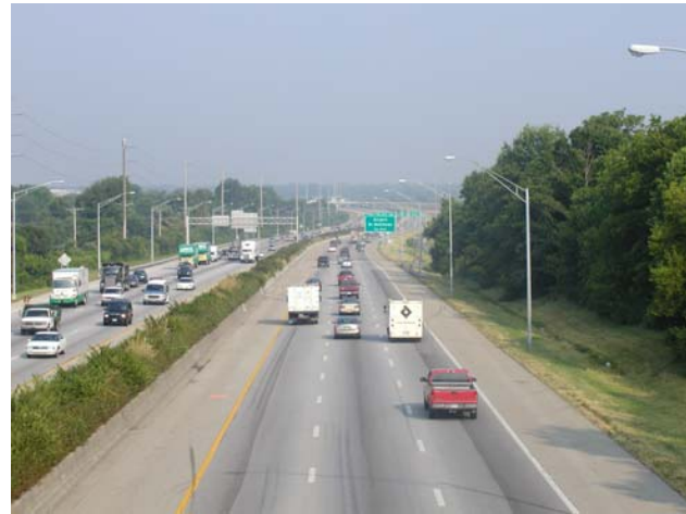
1 – Oxmoor Farm Road Bridge over I-64 Looking West
